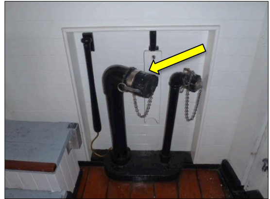
Sewage Shore Discharge Connection
