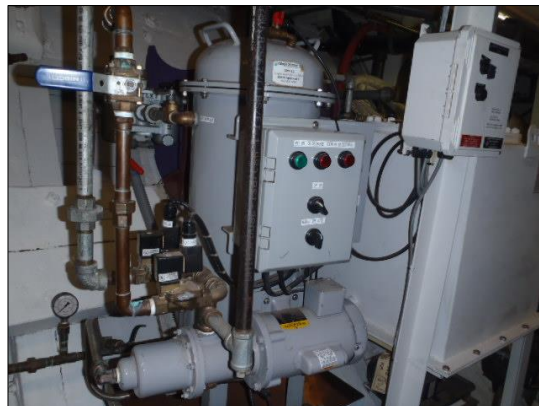
Oily Water Separator
