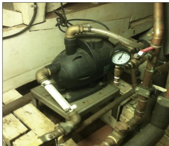
No. 1 Potable Water Pump
