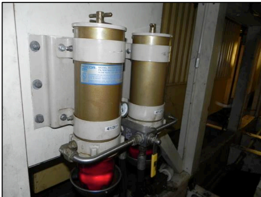
Boiler Fuel Filters (Lower Deck, E/R, Stbd side, FR 32)
