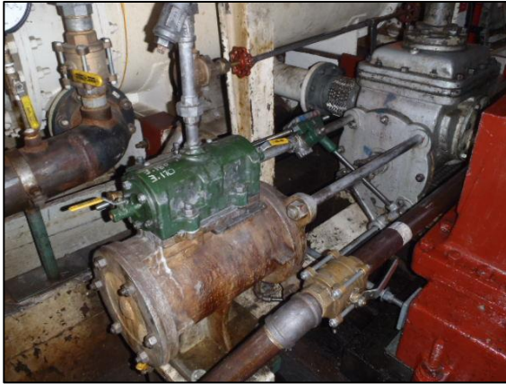
Main Air Pump (Lower Deck, E/R, Port side, FR 41)
