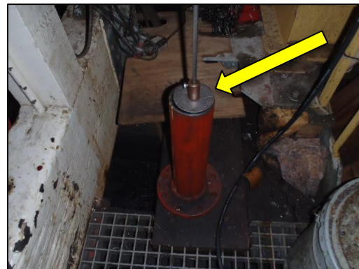
Torch used for manual firing (Emergency Operation Only)
