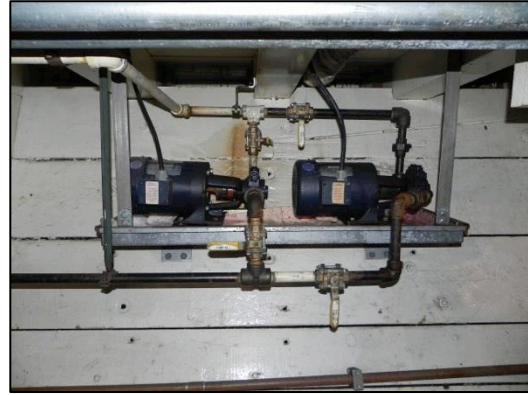
Electric Fuel Pumps (Lower Deck, E/R, Stbd side, FR 37)
